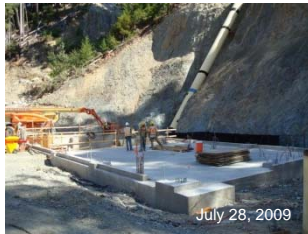
3. Building footings and concrete slab.
