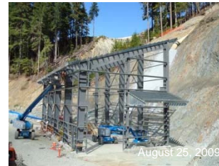
5. Construct steel building frame.
