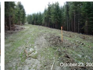
6. Backfill trench and seed.
