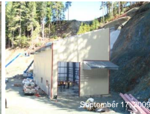
6. Install siding, roof, and windows.
