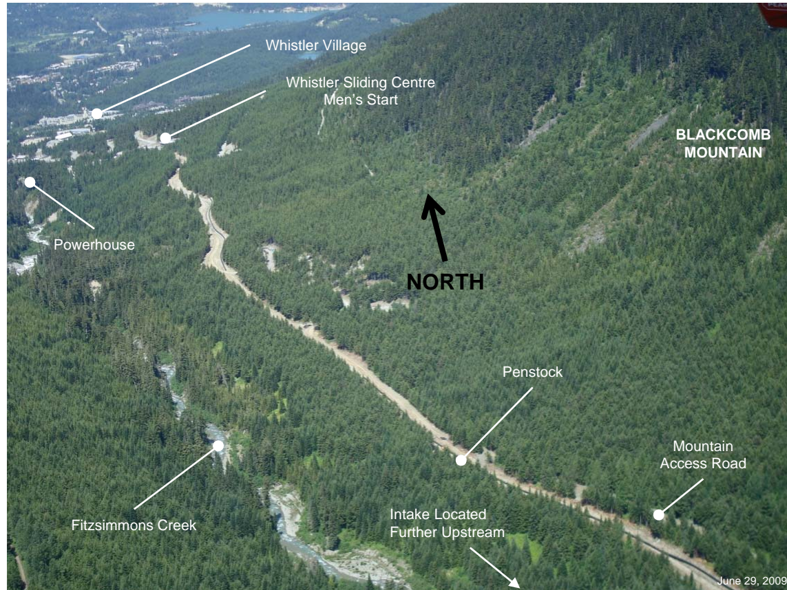
Penstock Route During Construction, Viewed from Peak-to-Peak Gondola.
