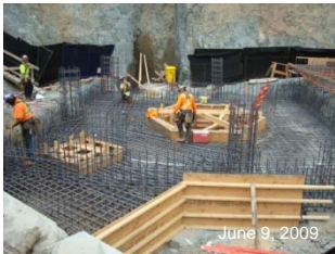
2. Rebar for turbine-generator floor.
