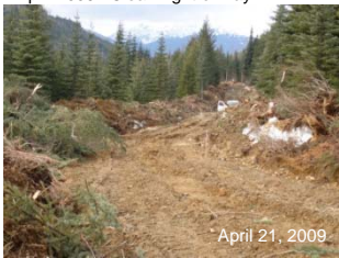
1. Penstock construction started in April 2009. Clear right of way.
