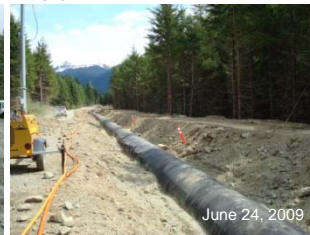
4. Fuse HDPE pipe lengths and place in trench.
