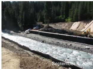
1. Intake construction started in October 2008. Excavate foundation.
