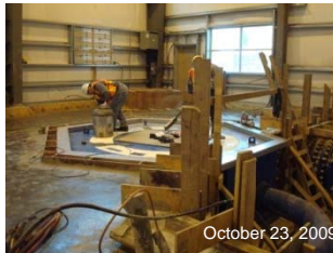
9. Concrete around manifold.
