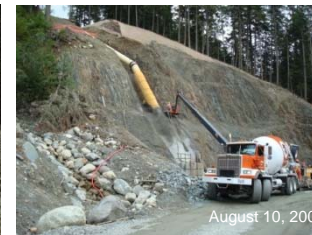
5. Grout on the steepest section down to the powerhouse.
