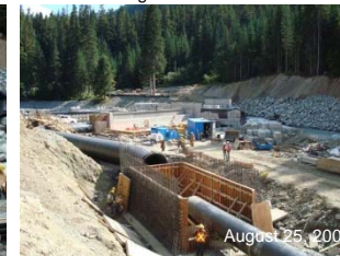
4. Construct regulation chamber.
