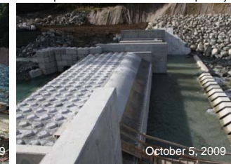
5. Completed Coanda screen and spillway.
