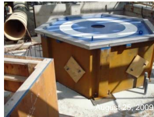
4. Turbine-generator housing.
