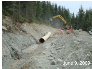
3. Steel pipe is lined, coated, placed and welded.
